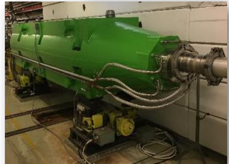
Assembly inside tunnel
